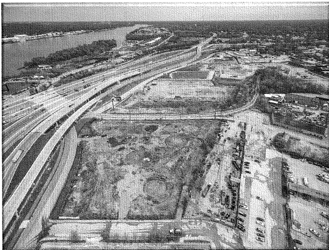
Photo 14: Louisville Soccer Complex, Construction Phase
